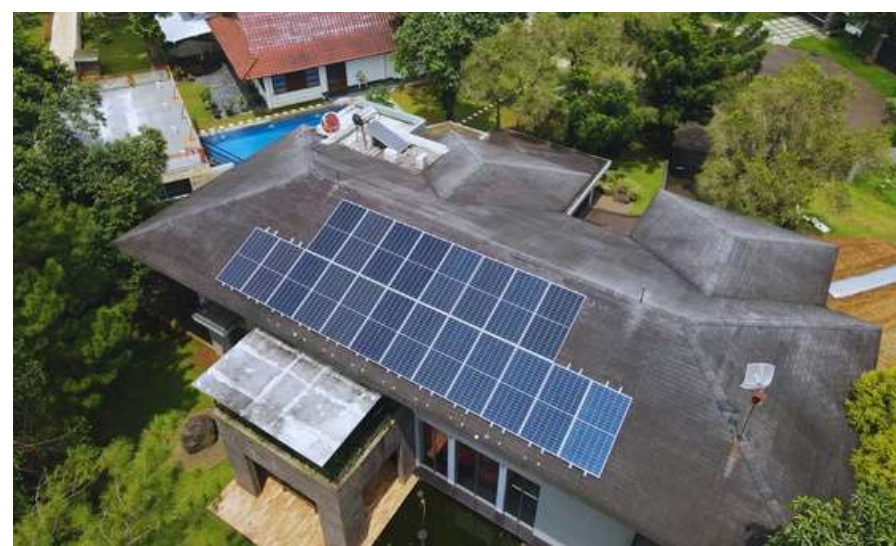
Bogor, Jawa Barat Capacity: 11 kWp
