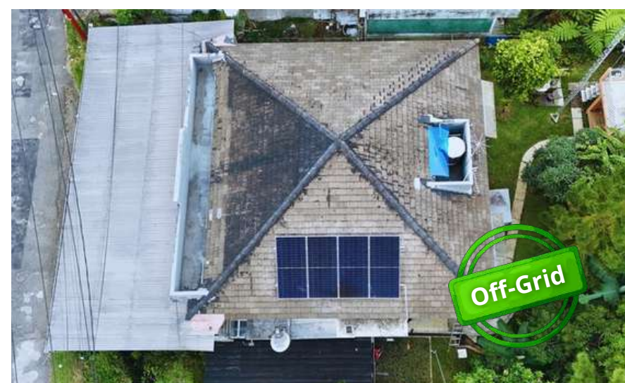
Bogor, Jawa Barat Capacity: 2.6 kWp
