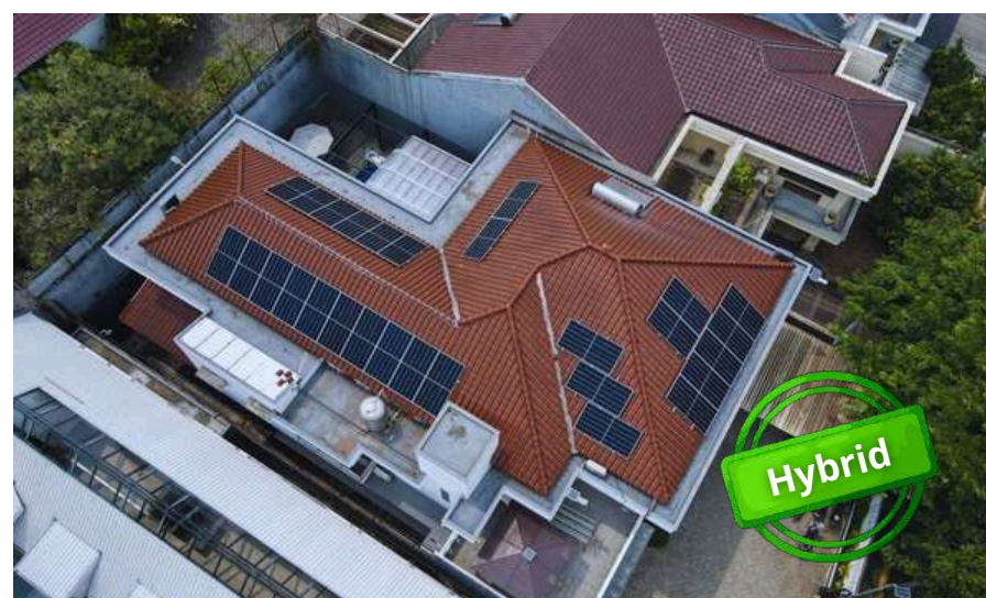
Bogor, Jawa Barat Capacity: 15.4 kWp
