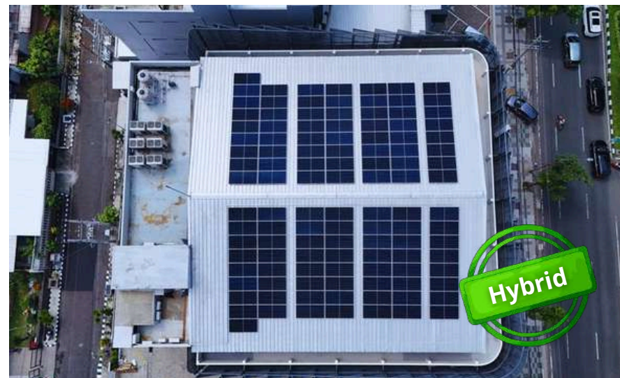
Surabaya, Jawa Timur Capacity: 74.1 kWp
