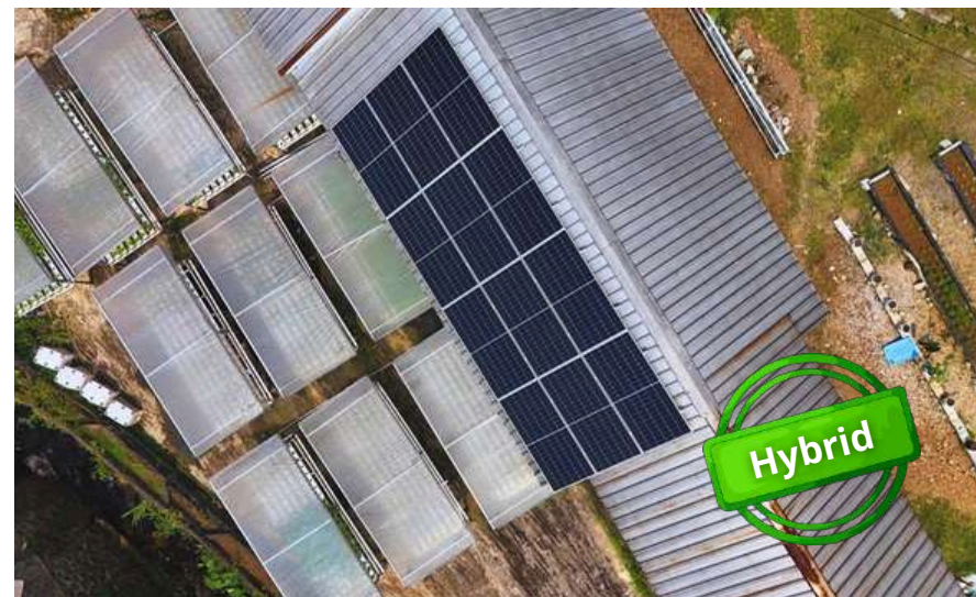
Bogor, Jawa Barat Capacity: 6.6 kWp
