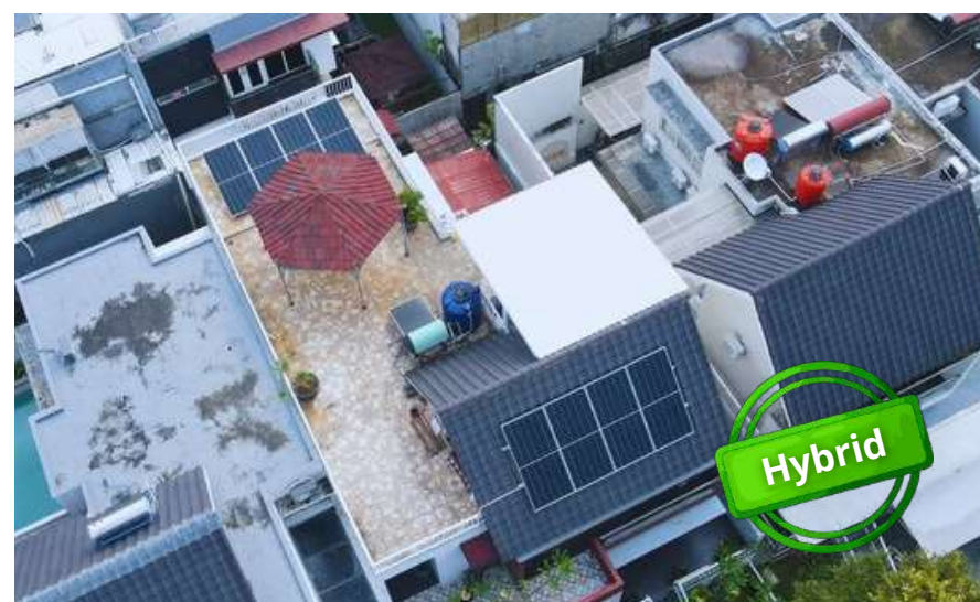
Bogor, Jawa Barat Capacity: 5.2 kWp
